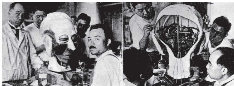
Figure 2. The construction of the rubber mask. Images appeared in Nishimura's article on the process of building Gakutensoku, published in Kagaku Chishiki (Science Knowledge)
