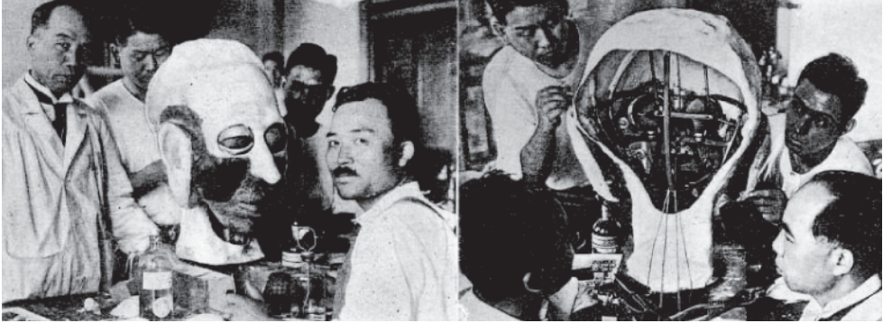
Figure 2. The construction of the rubber mask. Images appeared in Nishimura's article on the process of building Gakutensoku, published in Kagaku Chishki (Science Knowledge)
